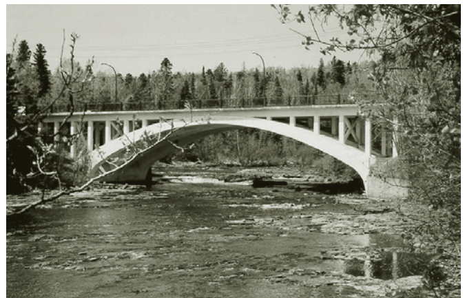
The Black Bay Bridge in the City of Thunder Bay is one of the first single spandrel, reinforced concrete bridges ever constructed. Constructed in 1912, this singular span bridge was designed to harmonize with the beauty and grandeur of the landscape. (Photo: Ministry of Culture)
