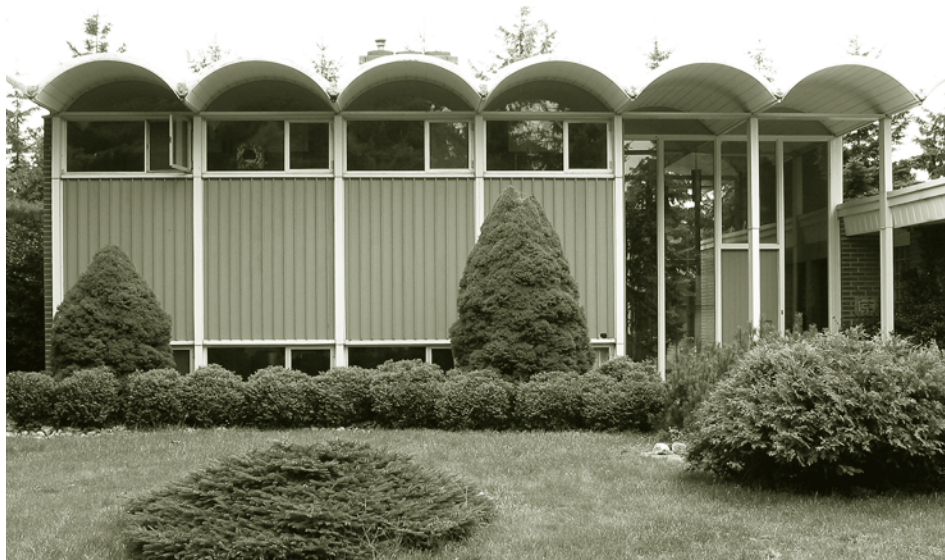
The Pagani House, built in 1961 and designed by architect Richard Pagani as his own home, is one of the best examples in Guelph of modern design. (Photo courtesy of Frank Hochstenbach)
