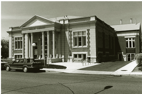
The new addition on the Woodstock Public Library respects the heritage value of the property. (Photo: Ministry of Culture)
